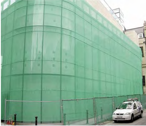
Figure 7.1.4: debris netting
