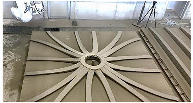
Fig. 7. Kloft et al. 2020 [39] imprinted 12cm wide SC3DP concrete ribs for structurally enhancing a thin-plated floor slab for a point-supported column consisting of an 8 cm thick concrete slab with dimensions of 4 m × 4 m.
