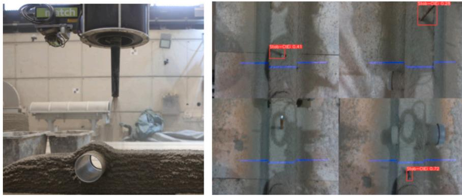
Fig. 15. Building installation integration during SC3DP at ITE TU BS with implemented process control height compensation (left). AI-based object detection and recognition using Intel RealSense data to ensure correct rebar positioning (right). Source: L. Lachmayer,
