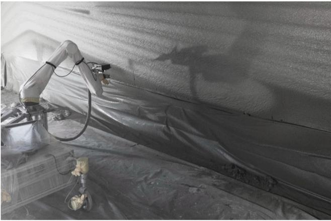
Fig. 5. Ercan Jenny et al. 2023 [37] introduced Robotic Plaster Spraying (RPS), a mobile, spray-based plaster printing technique.
