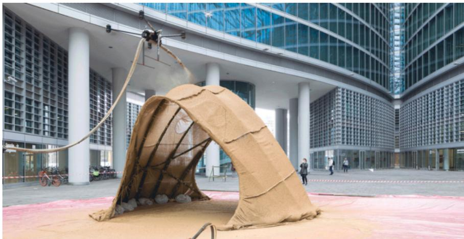
Fig. 6. Chaltiel et al. 2020 [38] demonstrated how a 2 m-wide drone with 50 cm legs and 20 min of flight autonomy tethered with a 20 m-long hose enabled the spraying of earthen mortar onto a fabric formwork.
