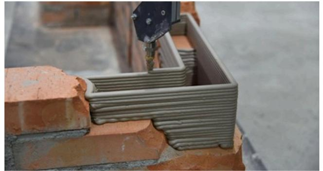
Fig. 3. Dielemans et al. 2024 [23] show the exemplary in situ 3DP of a replacement component within a brick assembly using surrogate material, employing a clay extrusion end-effector attached to the last link of a 6-degree-of-freedom (6DOF) robotic manipulator on a mobile robot platform.
