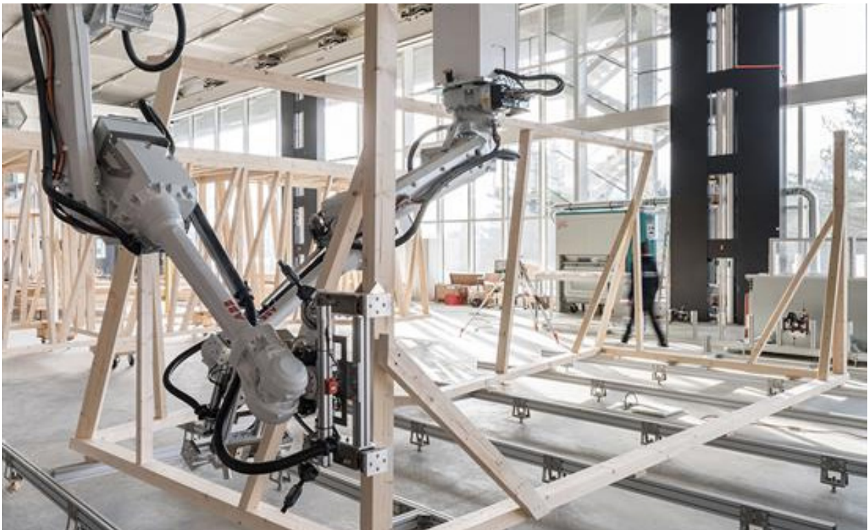
°Robotic timber assembly for prefabricated timber modules, GKR, ETH Zürich, 2018
