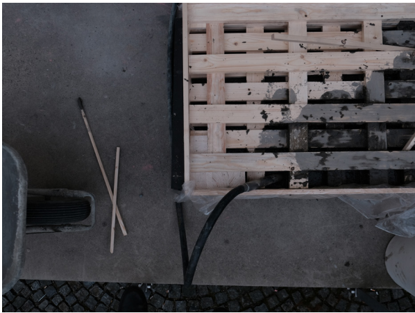
1:1 Mockup Casting Process
