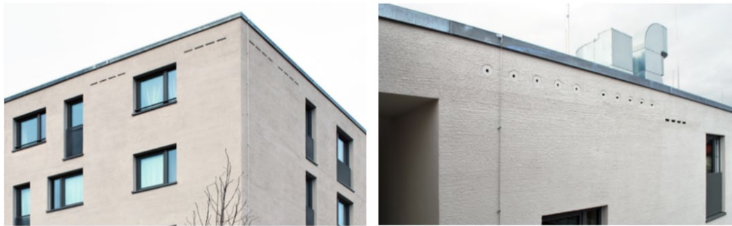
Figure 5: Integration of nests into buildings' facades, Weisser & Hauck
