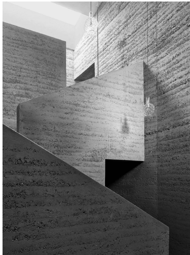
Fig. 44 Rammed earth surface.
