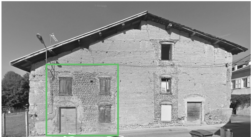
Fig. 19: Pisé building with fragments out of brick.
