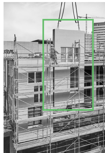
Fig. 29: Pre-mounted re-use windows.
