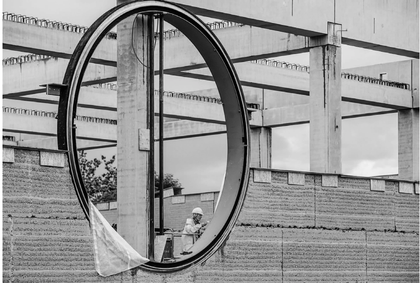
Fig. 31: Ricola Kräuterzentrum during construction.
