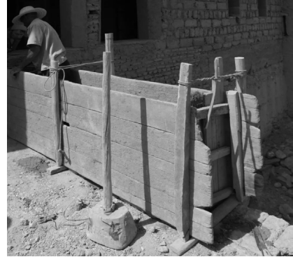
Fig. 2: Traditional rammed earth mould.
