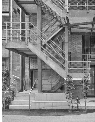
Fig. 21: Project K.118 re-used stair case
