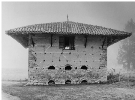
Fig. 3: Rammed earth building with beam holes.
