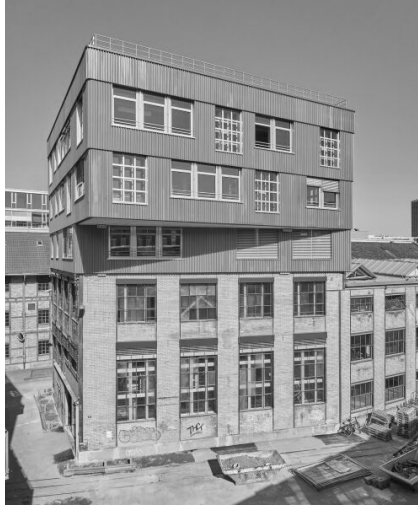
Fig. 20: Project K.118 by in situ Baubüro
