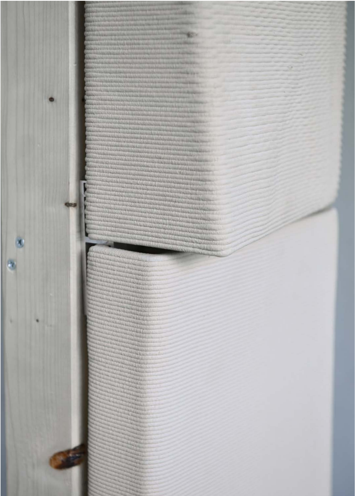
Entrance for the Bats at the Bat-Tile and Close-Up of the Microstructure 1:1
