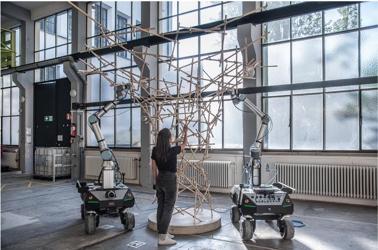
**Fig. 24** The final pavilion, consisting of 153 timber struts, was assembled by 17 people working in pairs, cooperating with two robots
