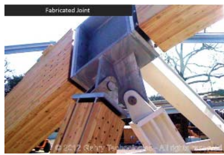
Figure 15: Joint - 3D modelling and fabricated (Gehry Technologies)
