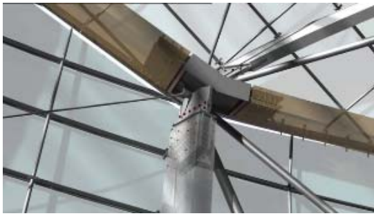
Figure 15: Joint - 3D modelling and fabricated (Gehry Technologies)
