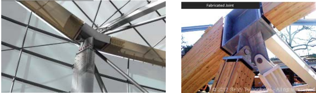
Figure 15: Joint - 3D modelling and fabricated (Gehry Technologies)
