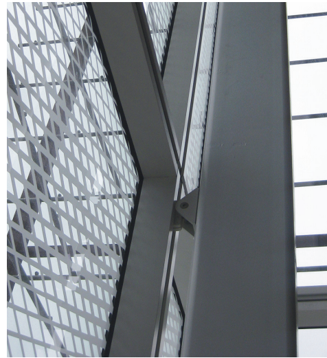
FIG. 4 Façade System Facts - Interior reveal frame profile houses custom designed lateral anchors providing visual separation from steel stick supports creating 2 thin and distinct façade planes.
