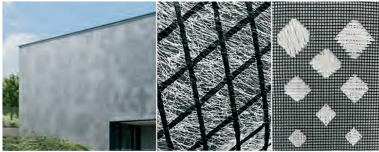
FIG. 12 Serge Ferrari textile façade creating patterns (left), Dimension-Polyant's X-Ply® Reinforced Monofilm reinforcement layers (center), weaving frit patterns on a textile substrate (right)
