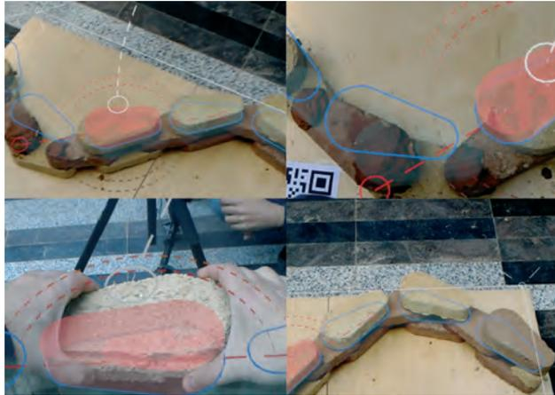
FIG. 5 HoloLens process. Active brick is highlighted in red
