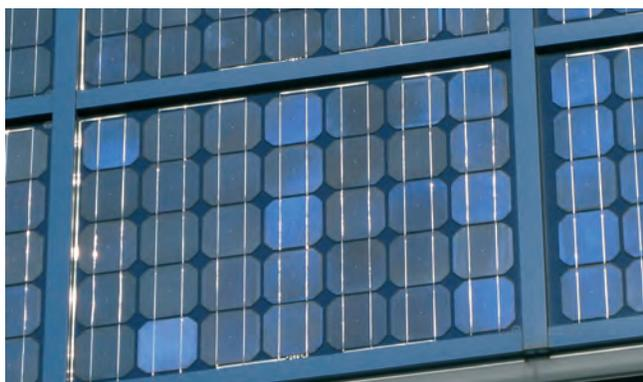
FIG. 5 Colour variation of cells that seemed to be of identical colour when not embedded.
