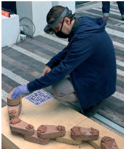
FIG. 7 Bricklaying with earth mortar
