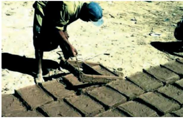
FIG. 1 Traditional production of adobe blocks in Saudi Arabia. Adobe mixture is manually pressed into wooden frames. Source: Mortada (2016)
