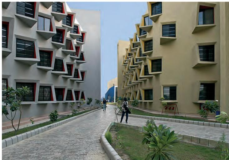
FIG. 8 Wedge-shaped bay window in the building. North-oriented windows overlooking gardens. Source: Sanjay Puri Architects
