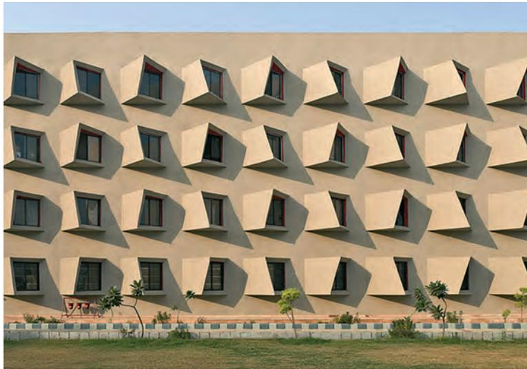
FIG. 12 North-oriented bay windows, The Street - Design process. Source: Sanjay Puri Architects
