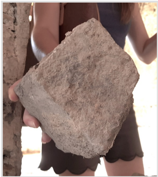
Opus Reticulatum a cubila of the facing used as a formwork, Villa Arianna, Stabiae, Italy
