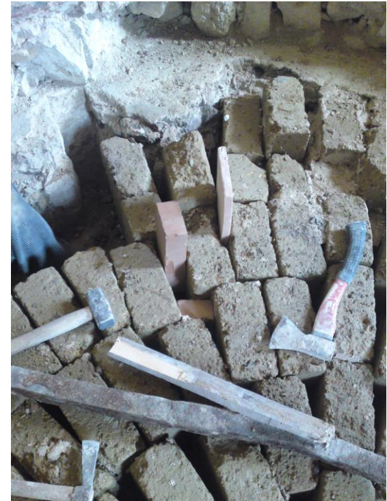
ROYAL PALACE OF NAPLES, RESTORATION WORKS
