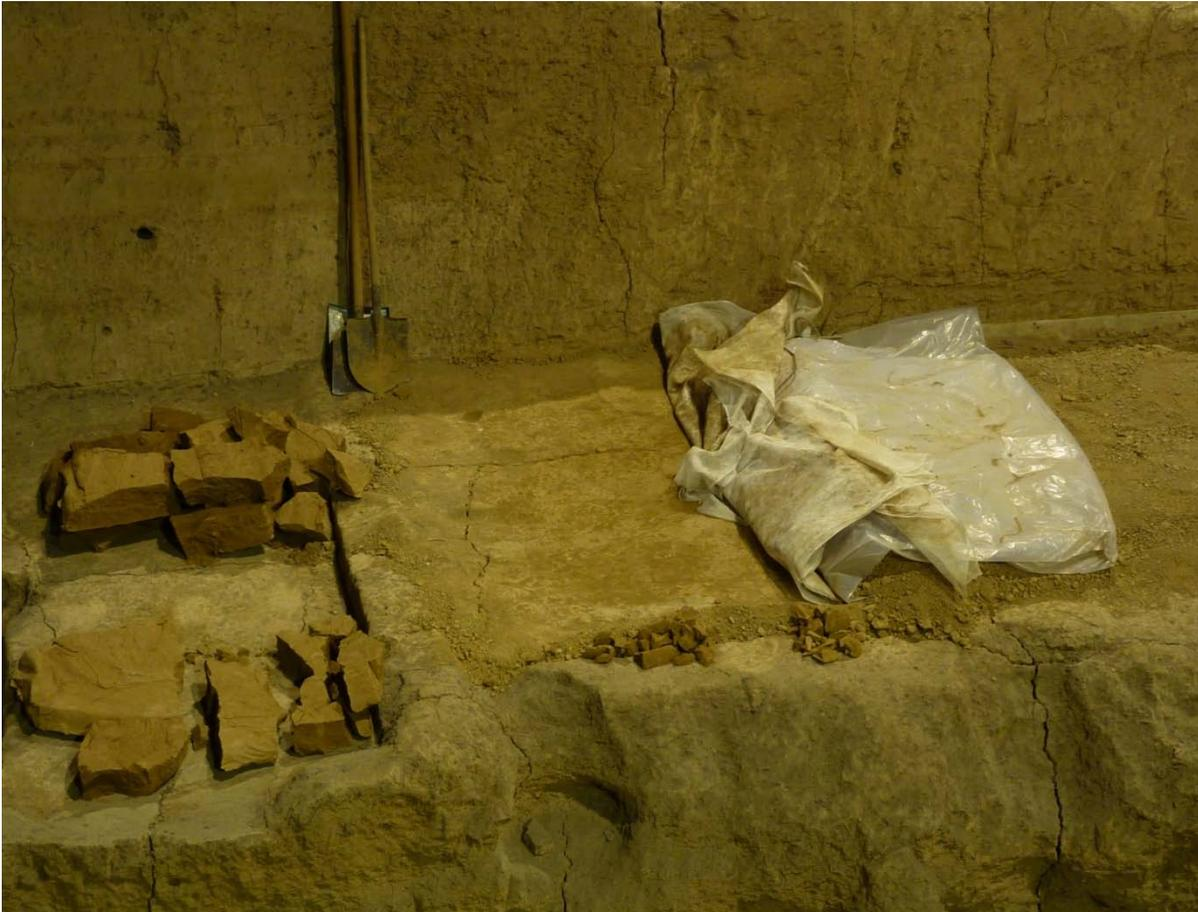
Figure 19: partly opened poultrice with uncovered removed plastic foil and protection fabric on the right side. Removed poultrice material on the left.
