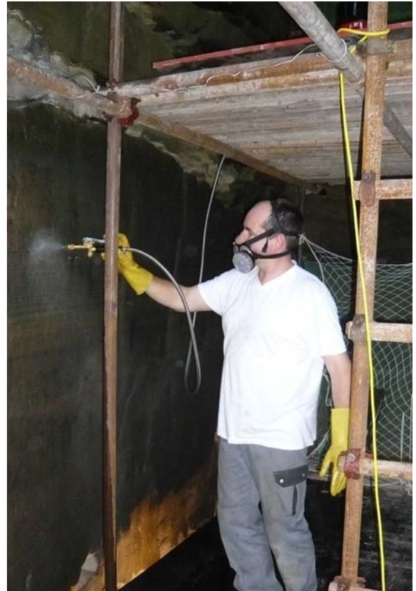
Fig. 32: Consolidation with spray coat method
