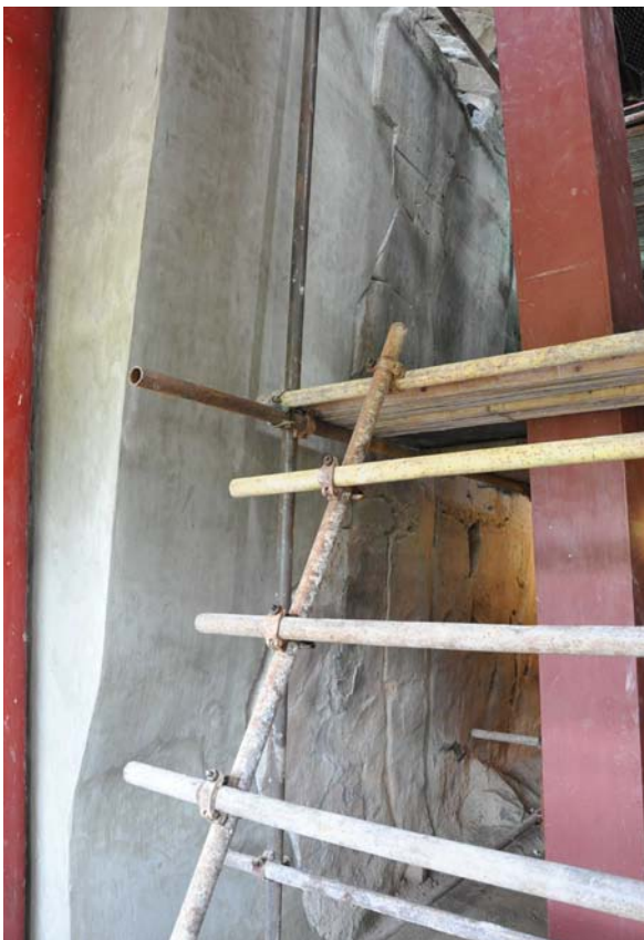
Fig. 6: New plaster on the East Wall
