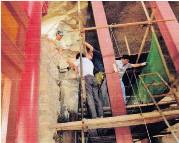
Fig.7/8: Drilling in the outer wall
