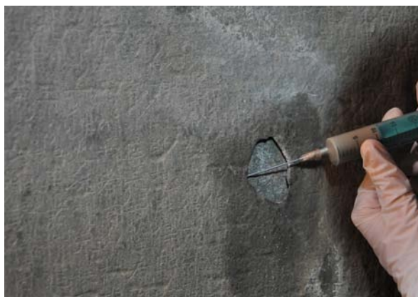
Fig. 27: Backfilling a void with open sides
