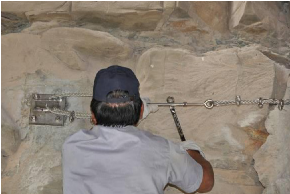
Fig. 11: Steel cable tensioning
