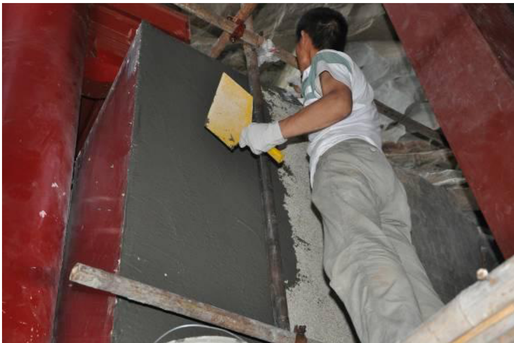
Fig. 27: Coating (repair mortar)
