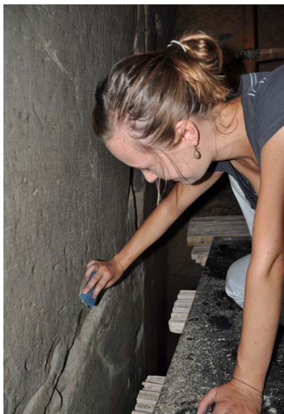
Fig. 22: Dry-cleaning of the wall with a Wish-up® cleaning sponge
