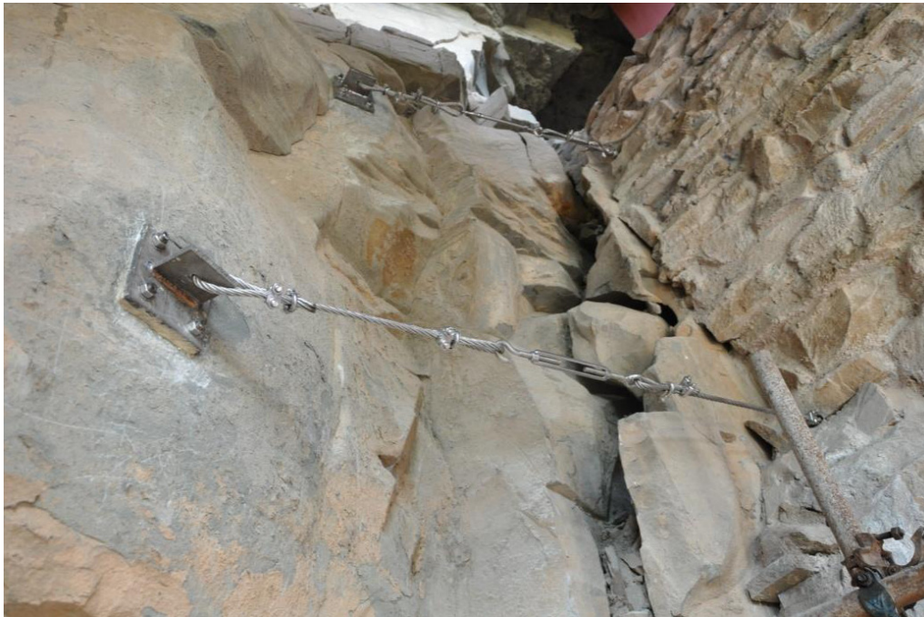
Fig. 12: Anchor joint outside
