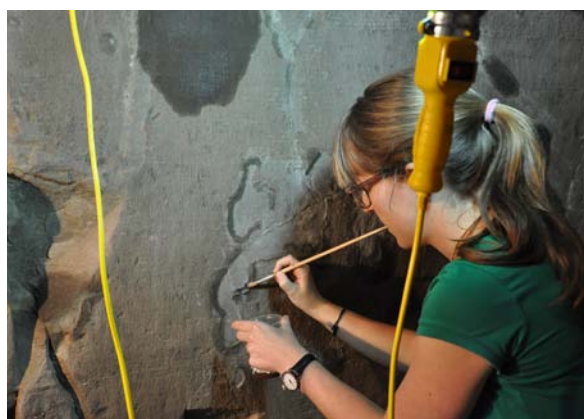
Fig. 30: Retouching the edges of bigger voids in the lower areas
