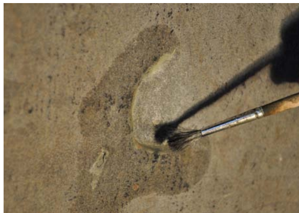
Fig. 29: Retouching the edges of an backfilled void after reworking the plaster
