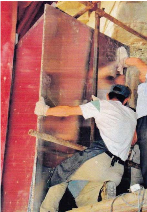
Fig. 15/16: Fixing the boards (honeycombed aluminum sheet)
