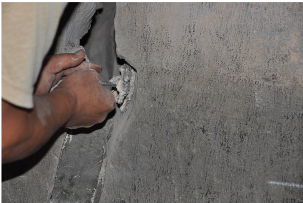
Fig. 29: Point connection by glue
