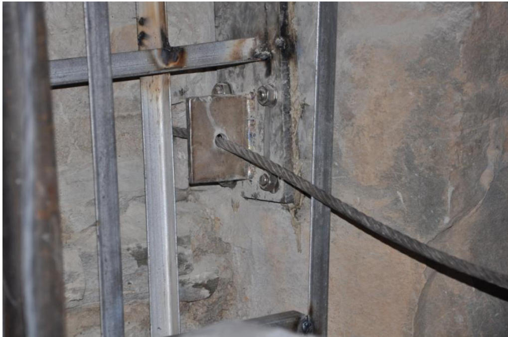
Fig. 9: Connect with steel plate
