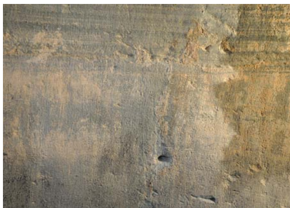
Fig. 20: Incrusted loam on the surfaces
