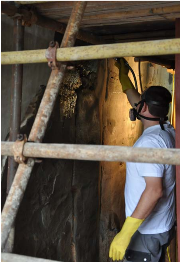
Fig. 31: Applying consolidation material (KSE OH) in spray coat method
