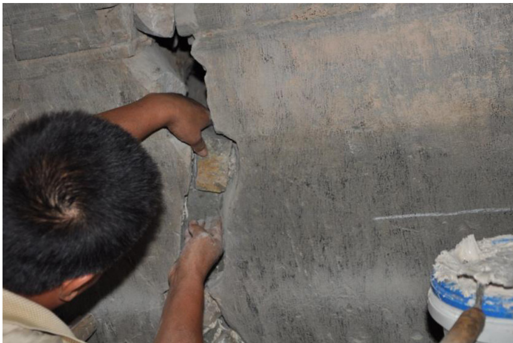
Fig. 28: Stone filling
