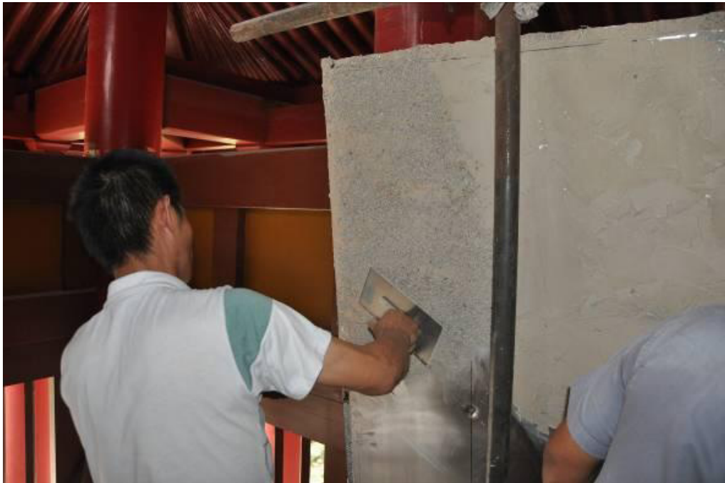
Fig. 26: Coating (sand processing)
