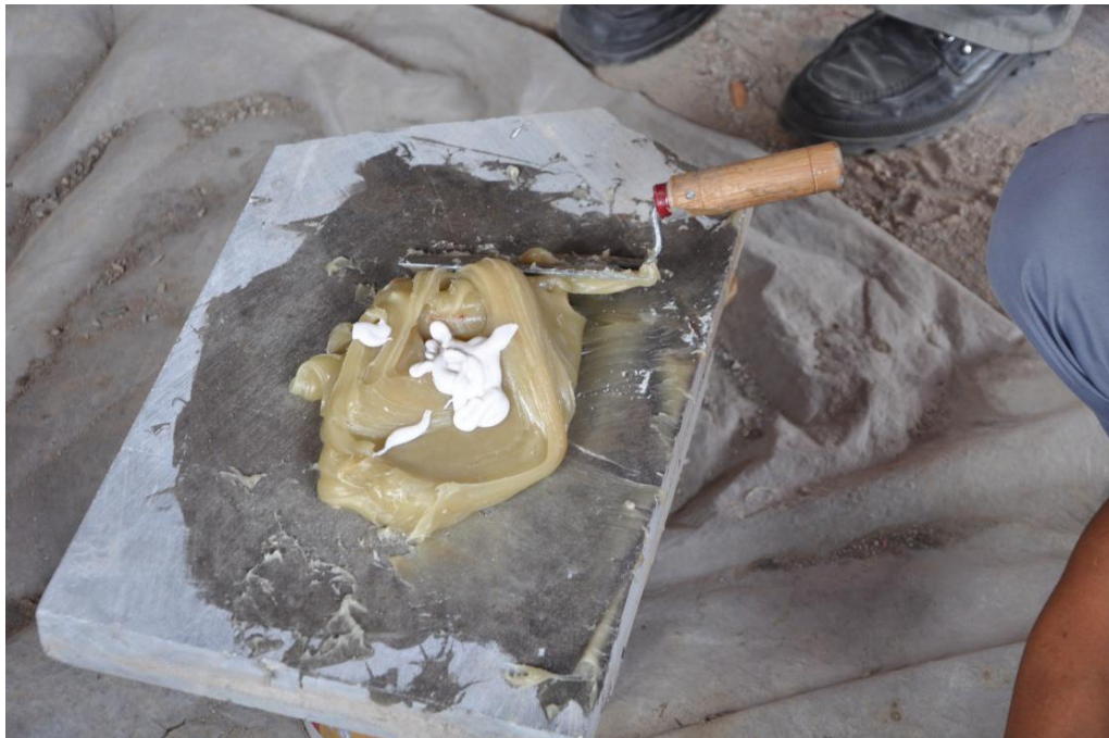
Fig. 24: Glue preparation
