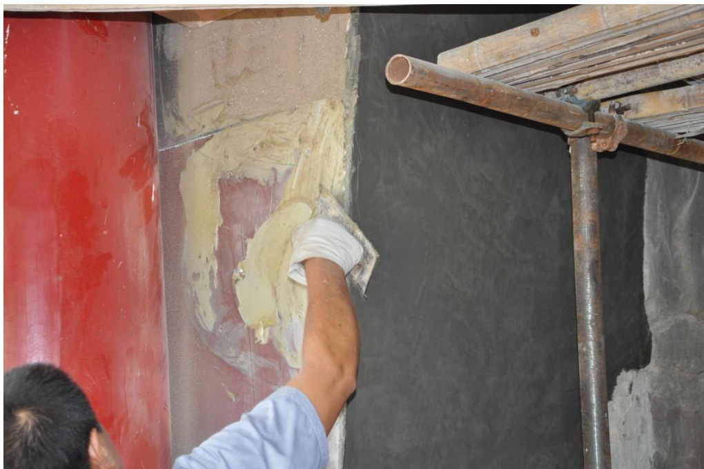
Fig. 25: Coating (glue)
