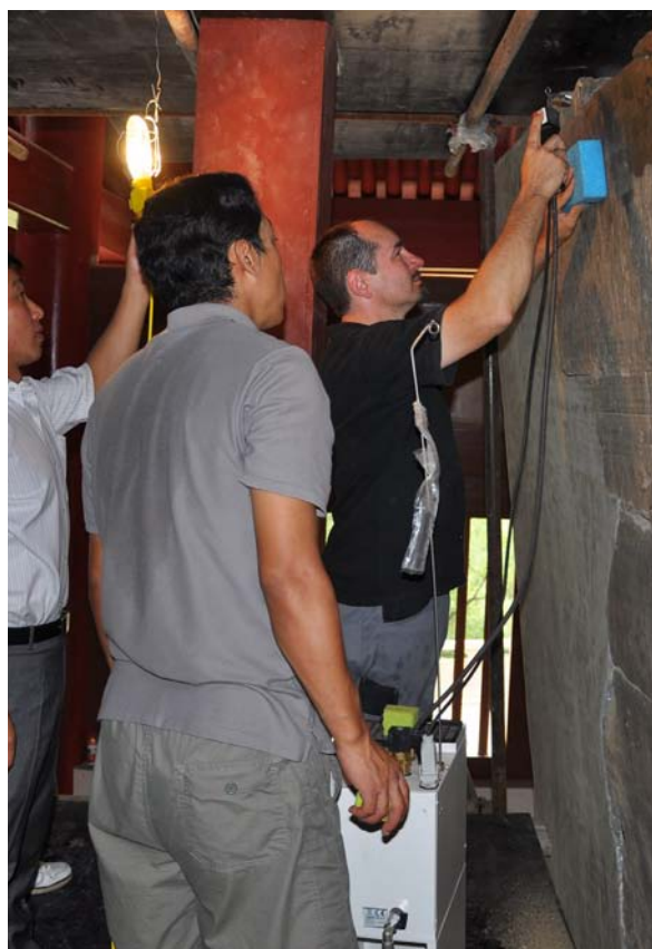
Fig. 23: Cleaning of the wall with water vapor
