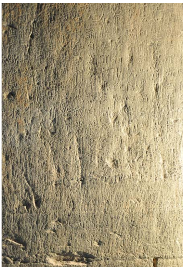
Fig. 24: Surface of the east wall after cleaning with sided light
