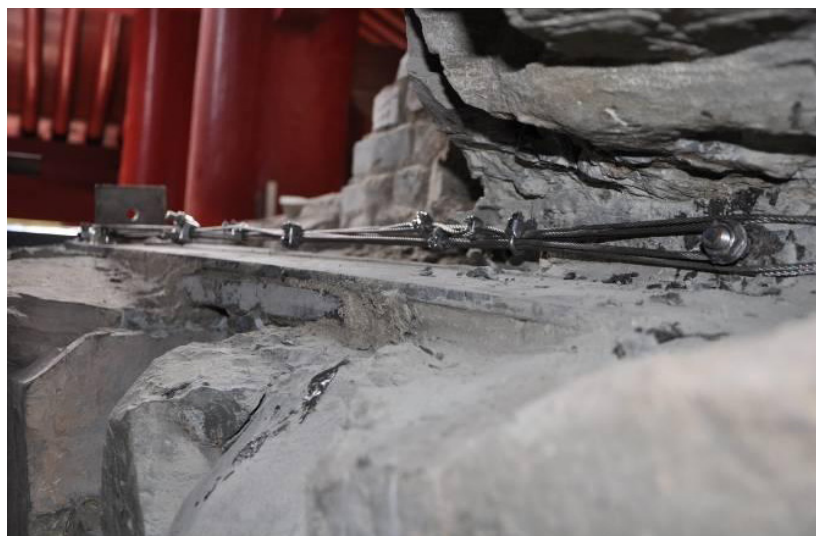
Fig. 18: Pull anchor finished (top)
