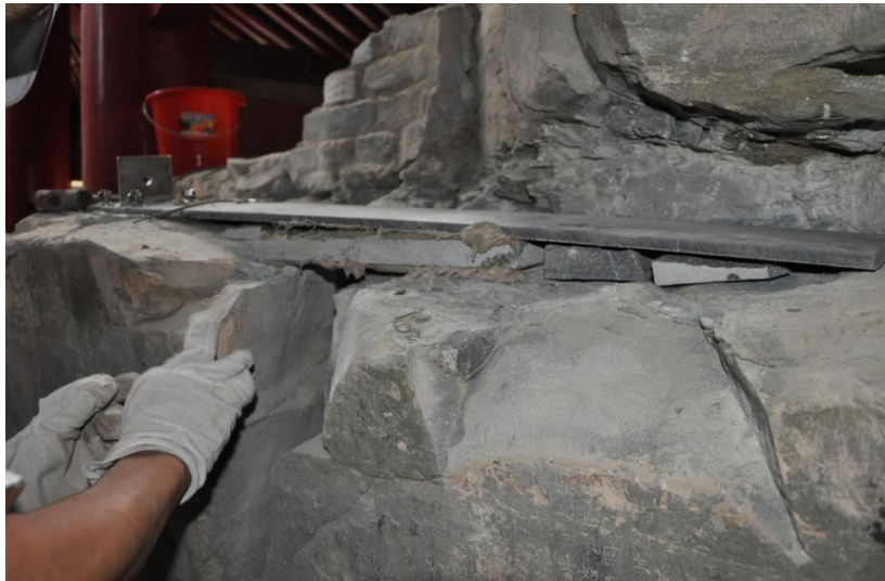
Fig. 15: Steel plate fixed (top)
