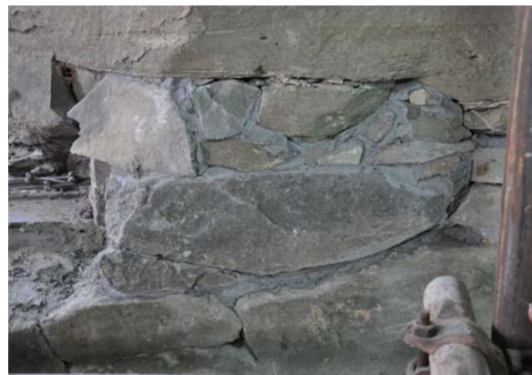
Fig. 17: Stabilisation of loose stones (with cement)
