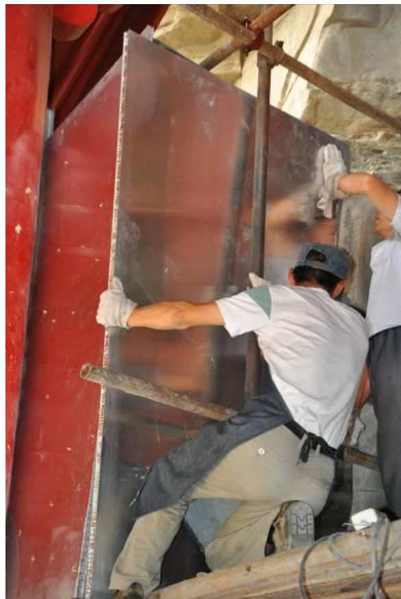
Fig. 23: Aluminum honeycomb panel fixed
