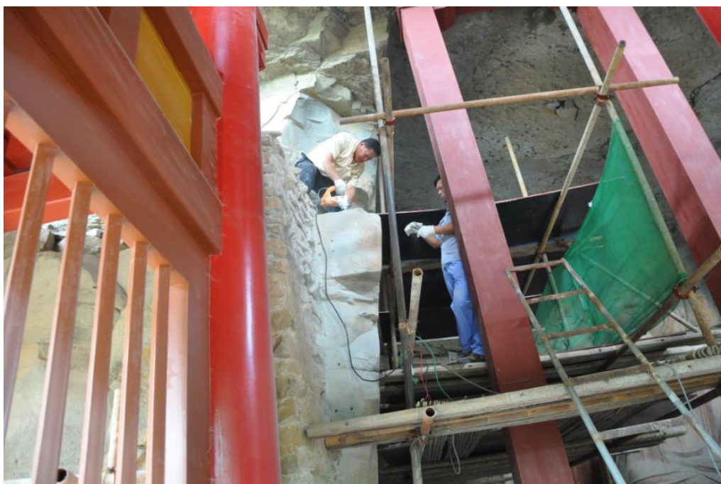
Fig. 13: Drilling (Rock top)
