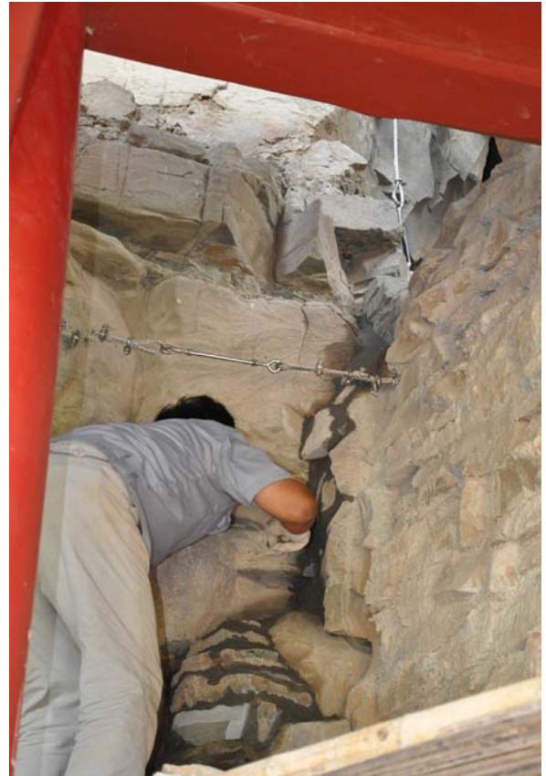
Fig. 7: Steel cables behind/above the East Wall
