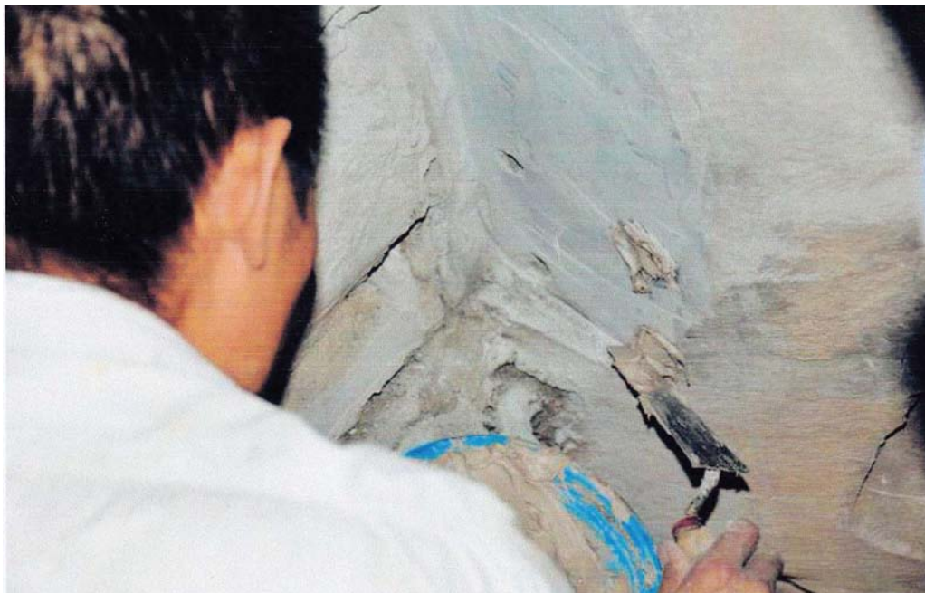
Fig.4: Filling with adhesive
