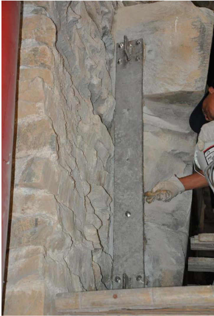
Fig. 6: Steel plate fixed
