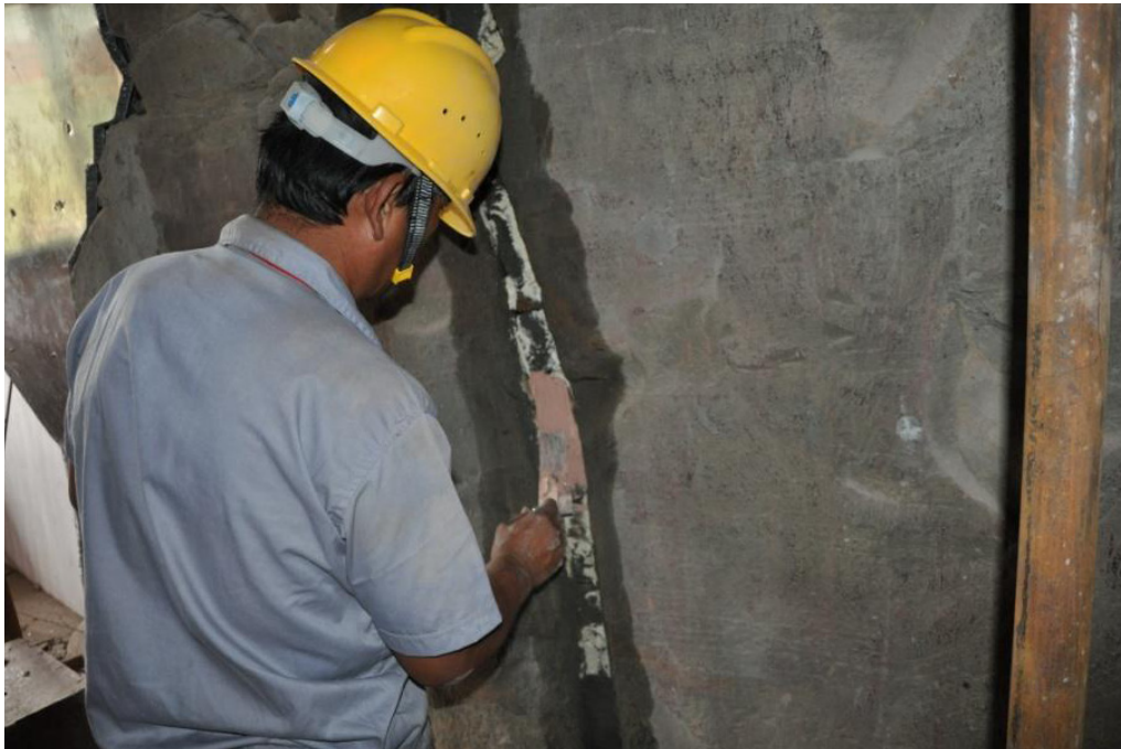
Fig. 30: Lime base mortar make level
