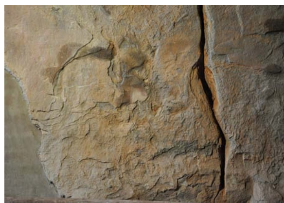
Fig. 26: Big voids and slaty cleavage near the floor of the east
