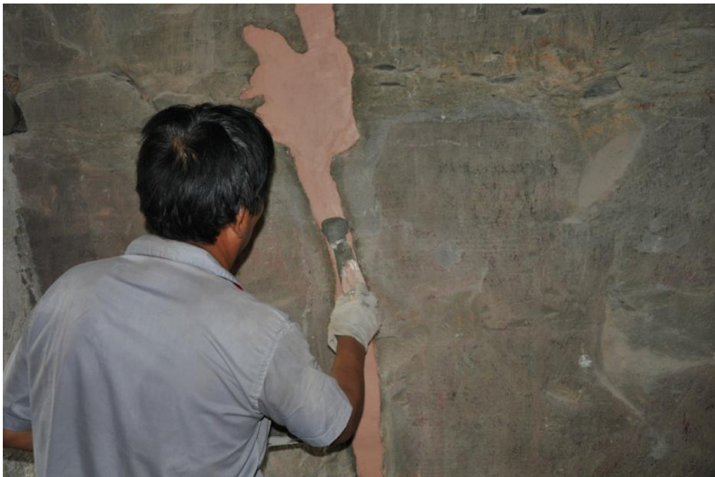
Fig. 31: Lime base mortar make level
