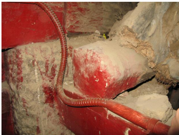
Fig. 11 Northern end of the lower pole lying on beam A and resting in a flat gap.
