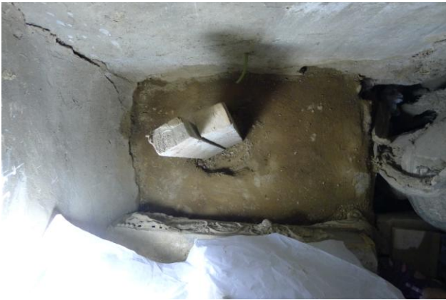
Fig. 89 The layer of coarse clay plaster with straw after being hit. By the wooden poles in the middle a whole is left for the re-inserting of the bodhisattva .
