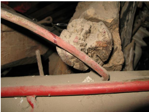
Fig. 9 Northern end of the upper pole lying on beam B and being secured with two iron pins.
