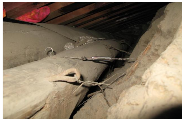
Fig. 74 The stainless steel wire is torn around the later inserted beam and a stainless steel turnbuckle holds the looped ends together.
