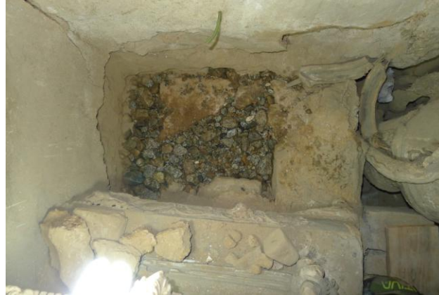
Fig. 88 The layer of stones is condensed by hitting.
