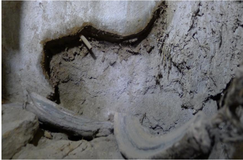
Fig. 104 The filling seals the edges of the plaster while grouting. An end of an injection tube is visible.
