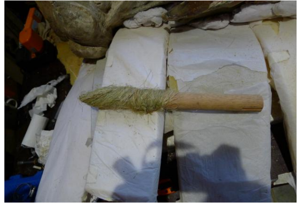
Fig. 94 The new wooden peg is wrapped with hemp fibres on that end that will extend into the plinth.
