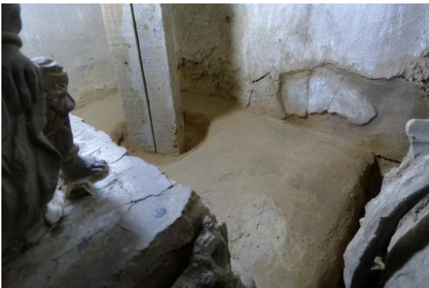
Fig. 91 The layer of fine clay plaster with hemp fibres after being hit. The surface of the new plaster is in level with the surface of a remnant of the original one (left front corner).
