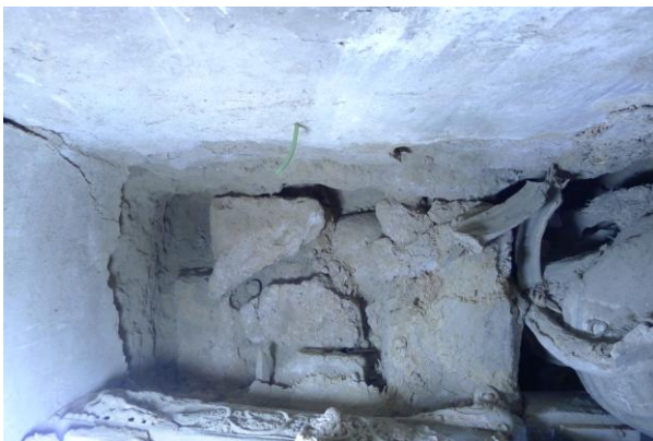
Fig. 85 After removing sand and debris the first firm bricks appeared.
