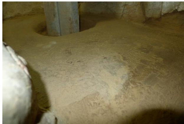
Fig. 92 The layer of fine clay plaster with hemp fibres after being hit. The remnant of the original clay plaster is visible in the front.
