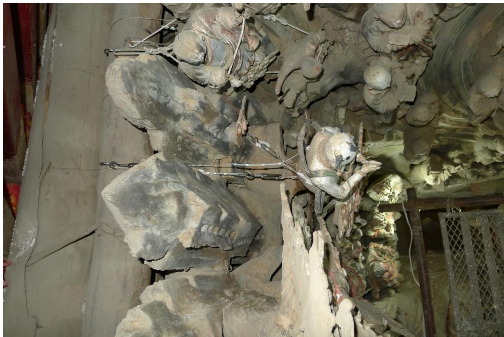
Fig. 81 The sudhana is reattached to his original position and is additionally secured to the beam of 1985.
