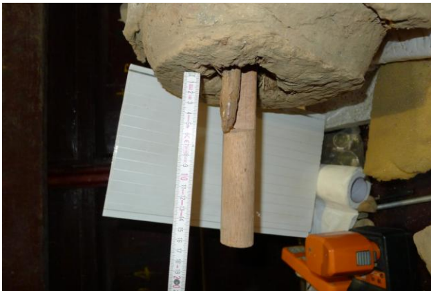
Fig. 95 The new pegs will extend 17.0 cm into the dais.
