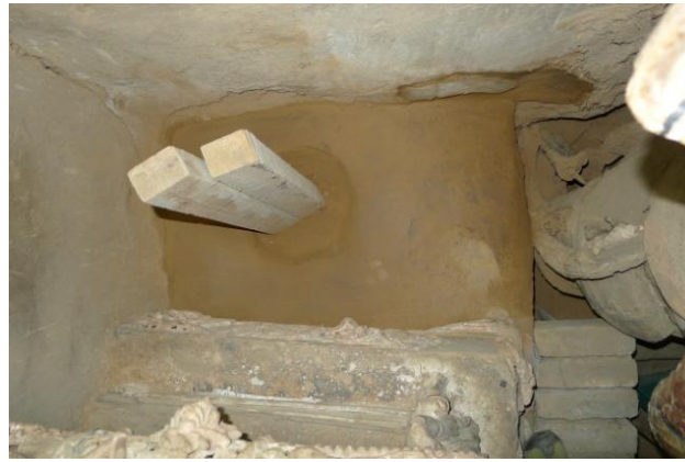
Fig. 90 The layer of fine clay plaster is applied onto the coarse clay plaster.
