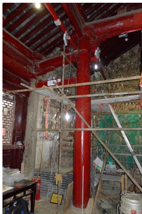
Fig. 8 Scaffold in front of ES wall.
