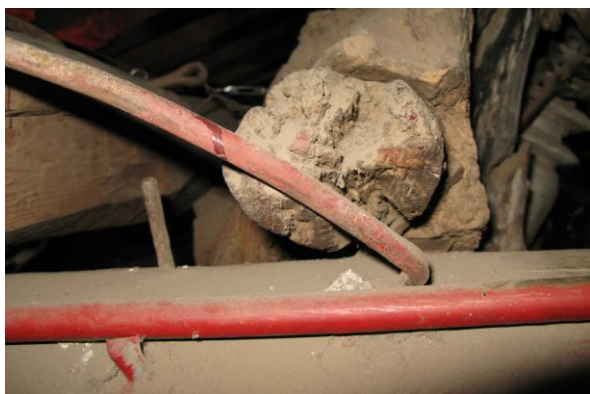
Fig. 52 The northern end of the upper pole rests not completely in the middle of the two iron pins.
