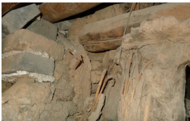
Fig. 53 The southern end of the upper pole does not rest on any element anymore but it hovers in the air.
