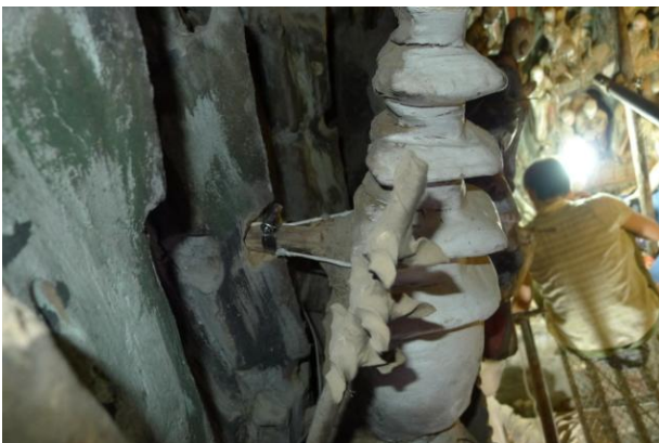
Fig. 73 The stainless steel clamp holds both parts of the encased wire together in order that the wire cannot cut into the surface.
