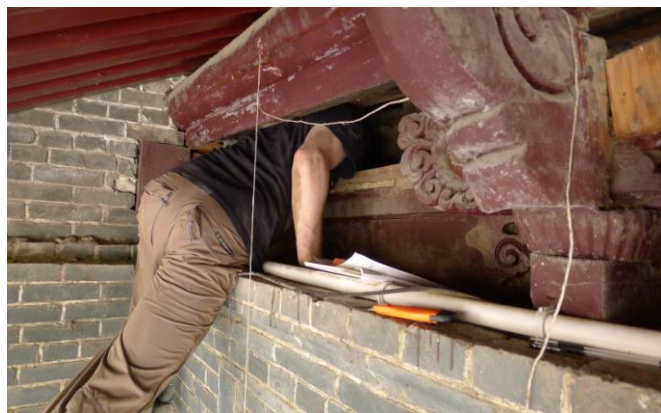
Fig. 7 Examination of the construction of the ES wall from the back after the removal of some panels.
