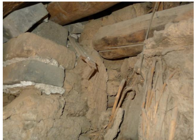
Fig. 10 Southern end of the upper pole hovering in the air.
