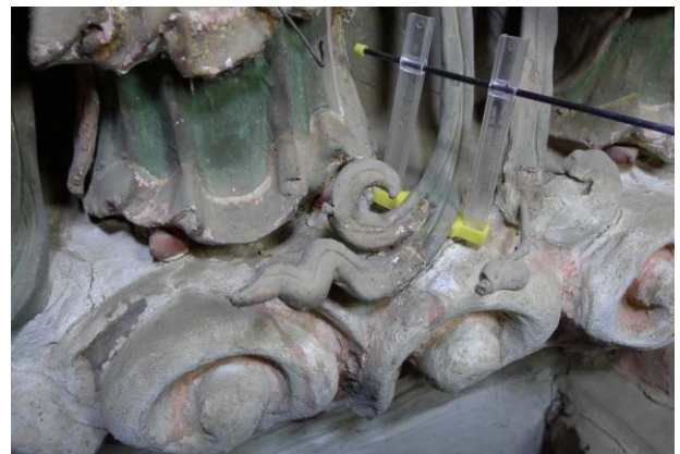
Fig. 100 Temporarily fixation with a clamp.
