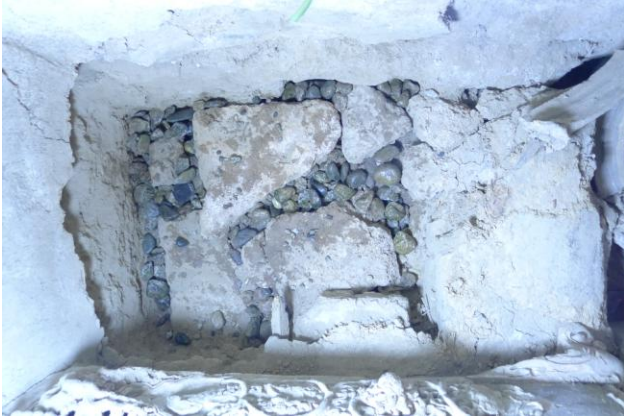
Fig. 87 A first layer of angled stones is filled in between the bricks.
