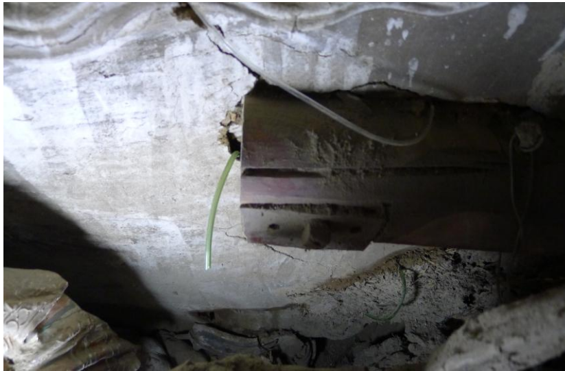
Fig. 105 Injection tube for grouting.
