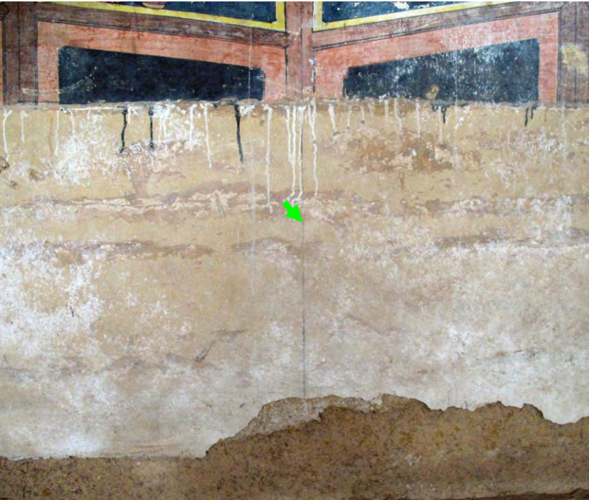
Fig. 79 Chalk line marking the centre of the pingfeng bei -painting or the vertical axis of the pedestal (green arrow). Runs from low viscose white ground, reddish and black paint at the upper edge of the lost pedestal.
