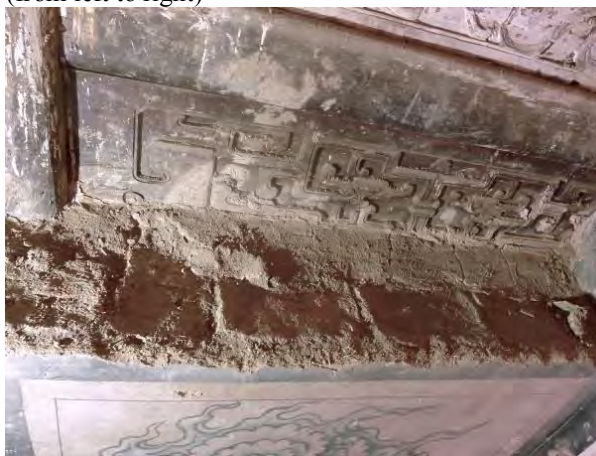
Fig. 77 Top edge of the yunqi xi -painting: Sequence of adobe bricks with one stretcher, one header, three stretchers (from left to right)
