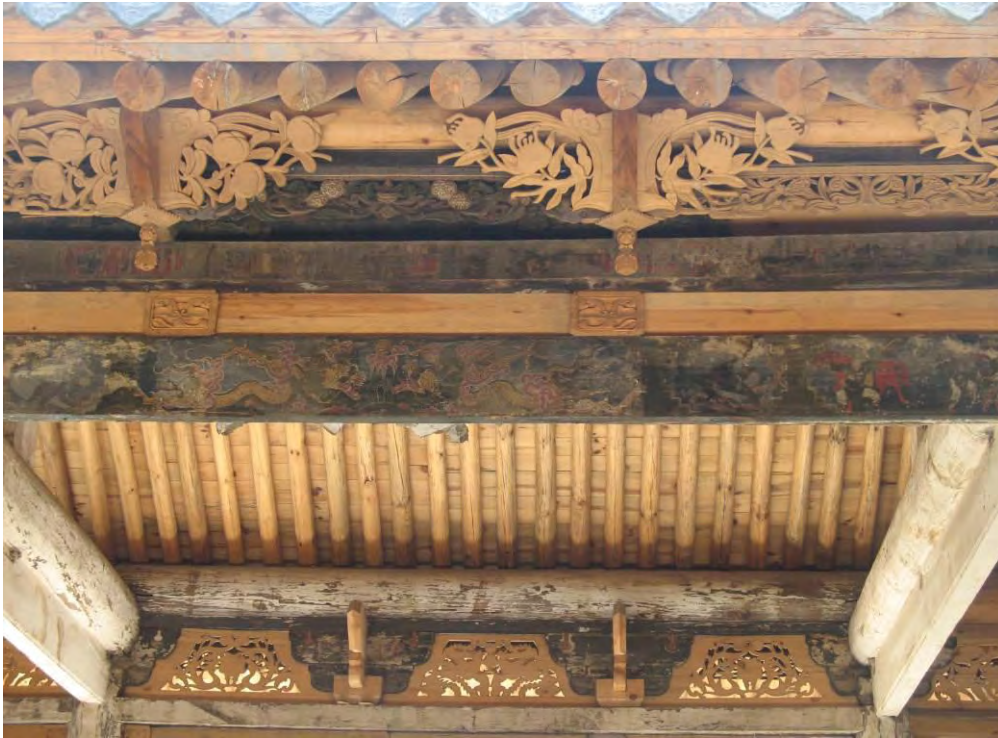
Fig. 19 Guodian, northern side (rear side), central bay. All original wooden elements are painted. Inside the hall traces of paintings can be recognised. Some parts are the beams are still covered with white-wash from the 1950's.
