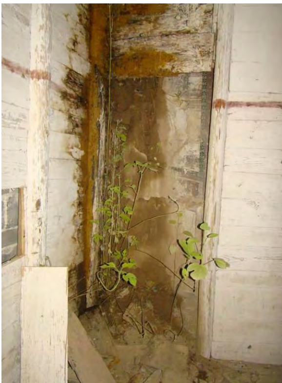
Fig. 55 Zhengdian, sanguo xi -wall during uncovering in 2006. The holes made by wooden pegs are closed with clay; runs of whitewash. [Shaanxi Institute for Conservation]
