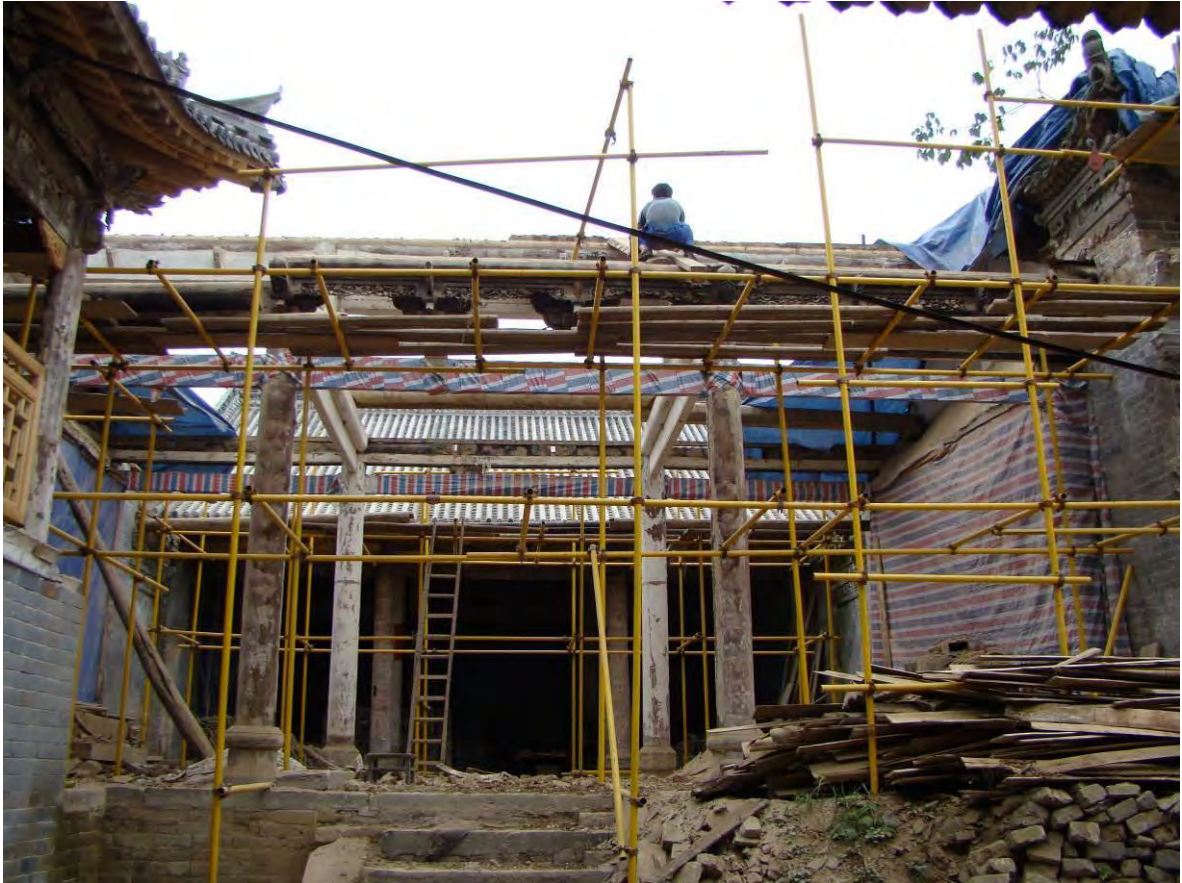
Fig. 67 Guodian during renewing of the roof [Jiang Bo]
