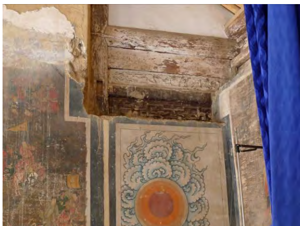
Fig. 72 Wooden construction above the yunqi xi , next to the sanguo xi
