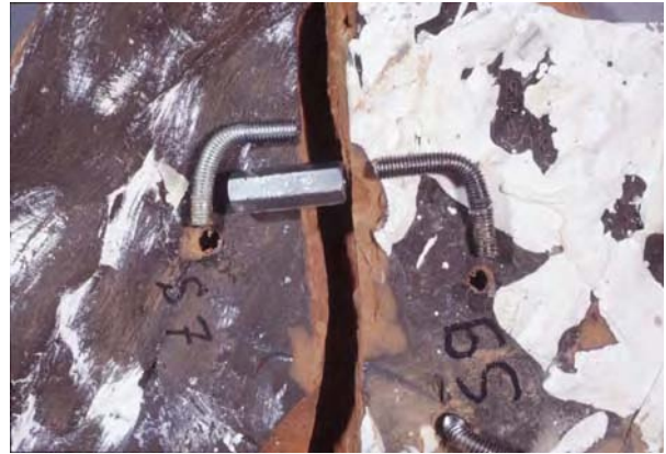
Screw cramp made for the assembling of the fragments.
