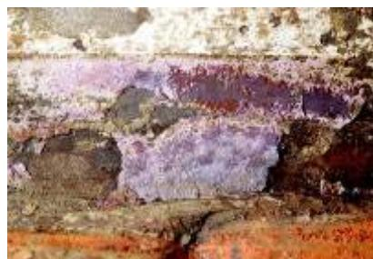
Fig. 23. after removal off the glossy material with acetone, Nov. 1, 2000
