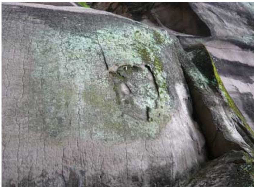
**Fig. 4:** Scaling as a reason of permanent moisture penetration
