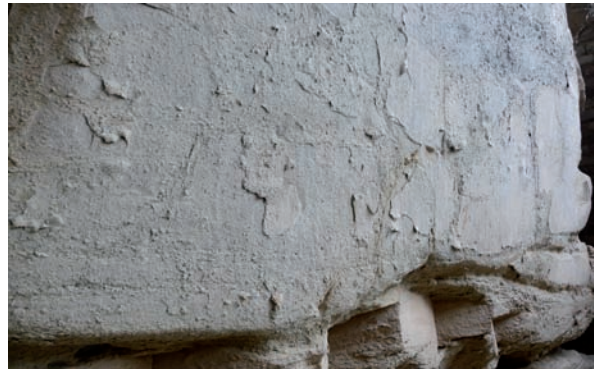
Abb. 16: Westwand, Detail obere Zone / Fig. 16: West wall, detail upper part
