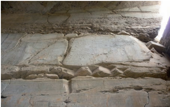
Abb. 15: Westwand, obere Zone / Fig. 15: West wall, upper part
