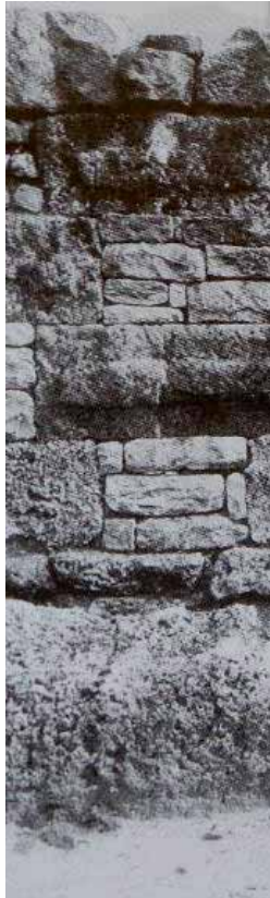
Chequer-work infilling, 3 rd c
