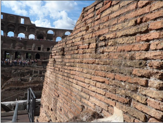
Left: Fig.11 - Opus testaceum, Colloseum, Rome (Rafail Evzonas)
