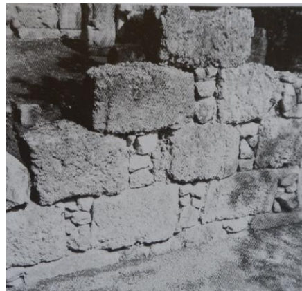
Right: Fig.5 - Bolsena, wall of chequer-work construction, 2nd century B.C. (Adams, 1994: 104, 119)
