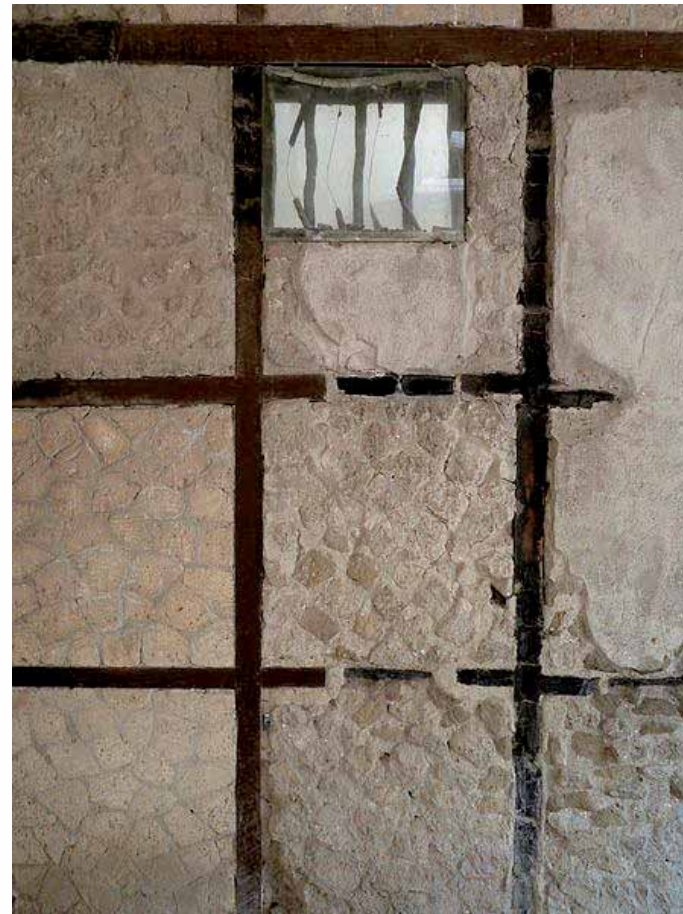
Herculaneum, opus craticium with rubbles as infilling
