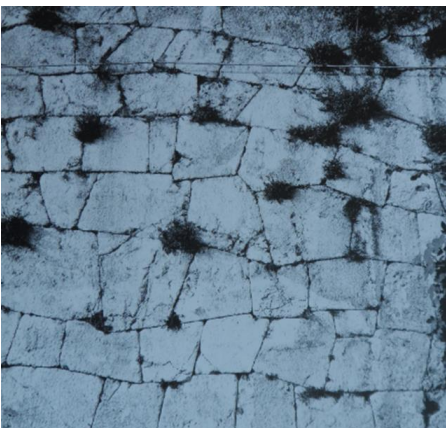
Left: Fig.4 - Opus siliceum, Pompeii, VIII.5.30
