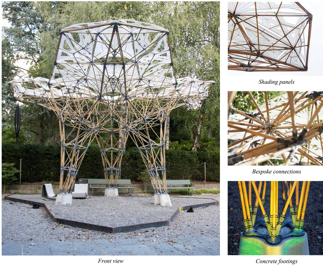
Figure 3: The Digital Bamboo at the *Bellerive Zentrum Architektur* in Zurich in 2020. [Photo: A. Jipa]
