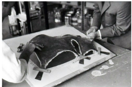
Figure 5. Heinz Isler, Studies on the form finding model of the Sicli project, 1968 (gta Archives, ETH Zürich).
